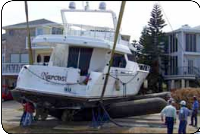
Narcosis was blocked briefly while the slings were lowered and the two spreaders and bridles rigged in preparation for picking up the full weight of the vessel.
