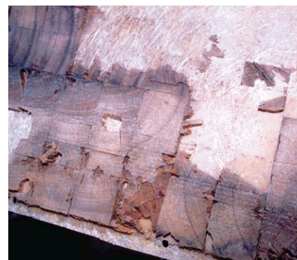
Water that leaks into the core can eventually cause rot.
